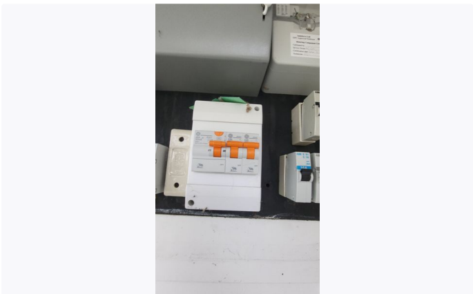
Ref #30 - modern RCD installed
