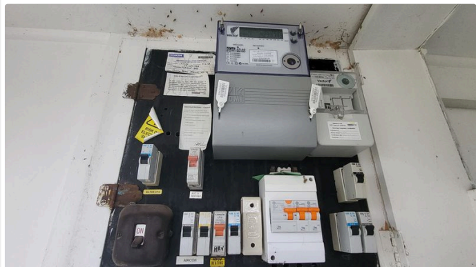
Ref #30 - Main board; mixed morden breakers installed
