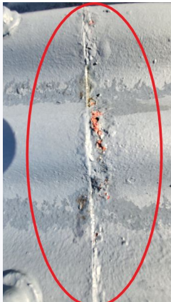
Ref #10.3 - Some oxidation or rust is visible in the laps joins, and some historic repa
