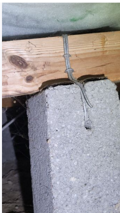
Ref #13 - Crawl Space example and reference photos; pile attachment method
