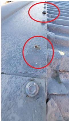
Ref #10.5 - Some loose or missing lead heads
