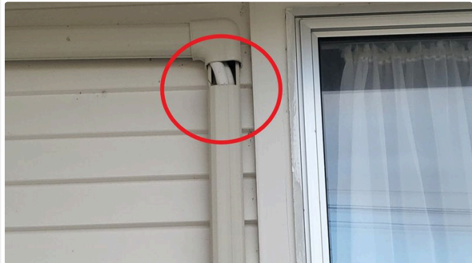
Ref #28.4 - ducting has come loose, minor maintained required;
