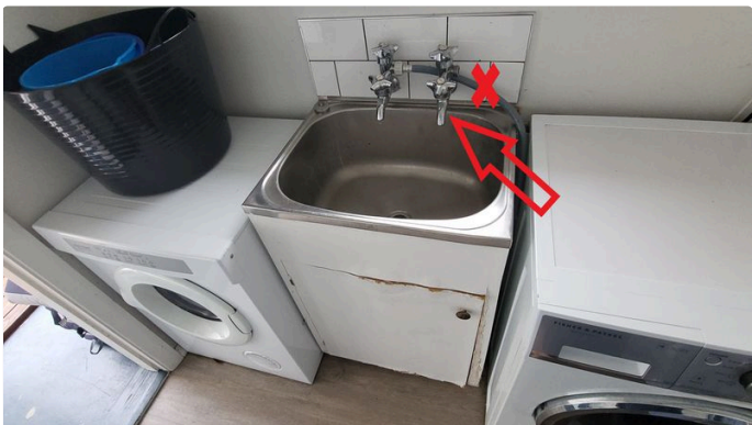
Ref #22.6 - loose tapware, no hot water from the faucet
