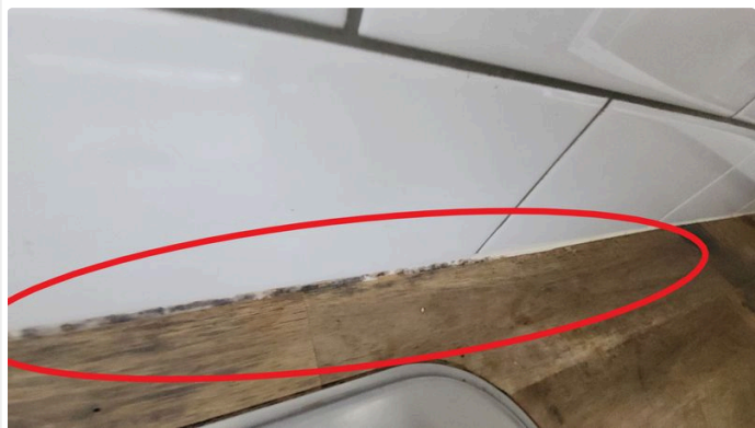
Ref #17.1 - Areas of mould growing in the silicone sealer, consider re-sealing for heal
