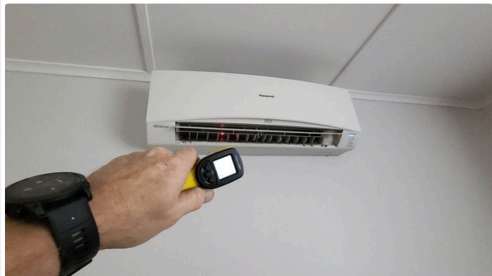
Ref #25.7 - The heat pump operated satisfactorily
