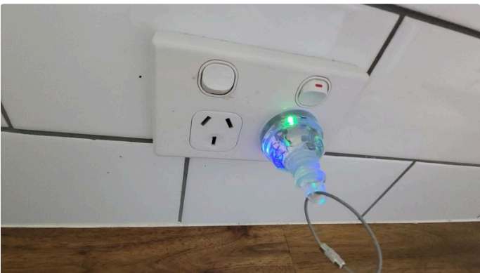
Ref #30 - Sockets polarity and earth have been checked
