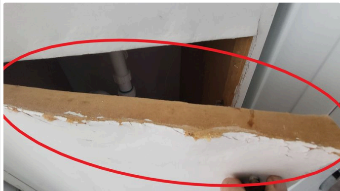
Ref #22.6 - puffy MDF, water damage
