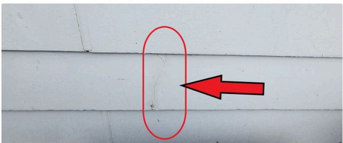
Ref # 8.1 - Repair or seal cracks in weatherboard
