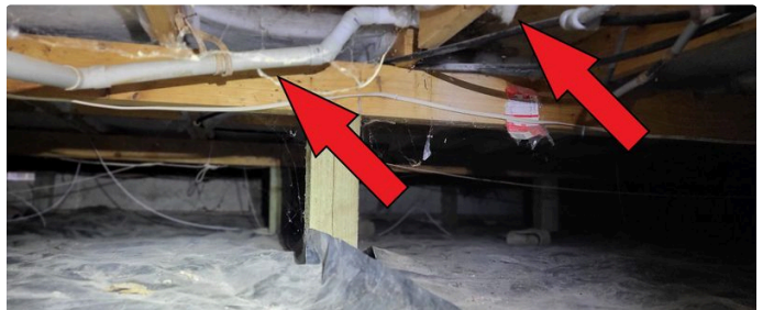
Ref # 13.14 - No S trap installed in the shower
