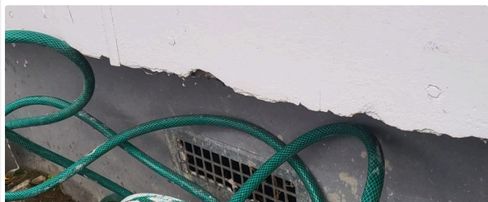
Ref # 8.1 - Chipped weatherboard in places
