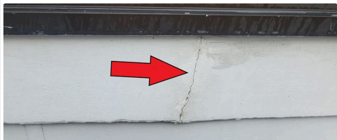
Ref # 8.1 - Repair or seal cracks in weatherboard
