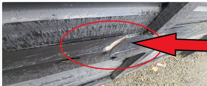
Ref # 7.4 - Timber break in the fence rail
