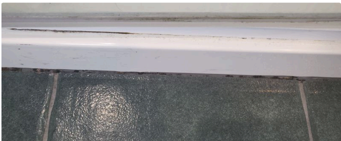
Ref #18 - moldy silicone , loose grout
