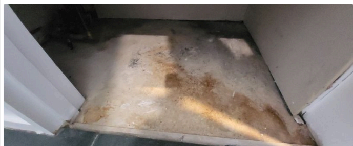
Ref # 15.5 - historic water staining and minor damage to the chipboard flooring
