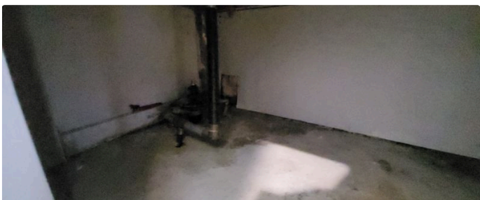
Ref # 15.5 - historic water staining and minor damage to the chipboard flooring
